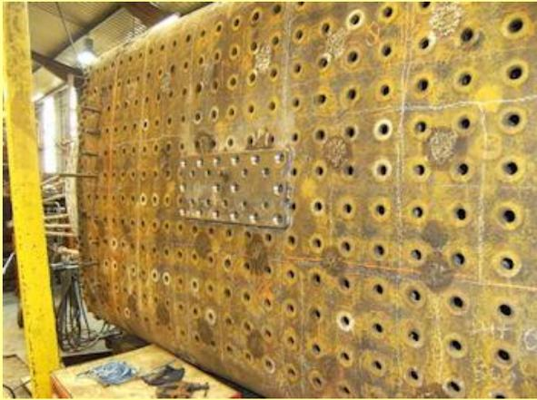
29/05/2013 - patch welder to the top of the outer firebox covering the aperture for the LMS safety valves fitted to the 8F boiler.
