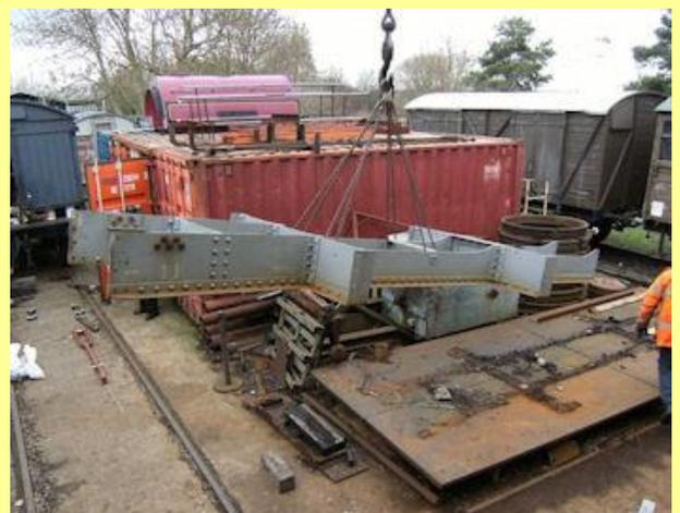
16/02/2013 - moving the ladder frame from the steel base plate, initially to enable shaping of cab roof, but also in readiness for despatch to Pontefract.
