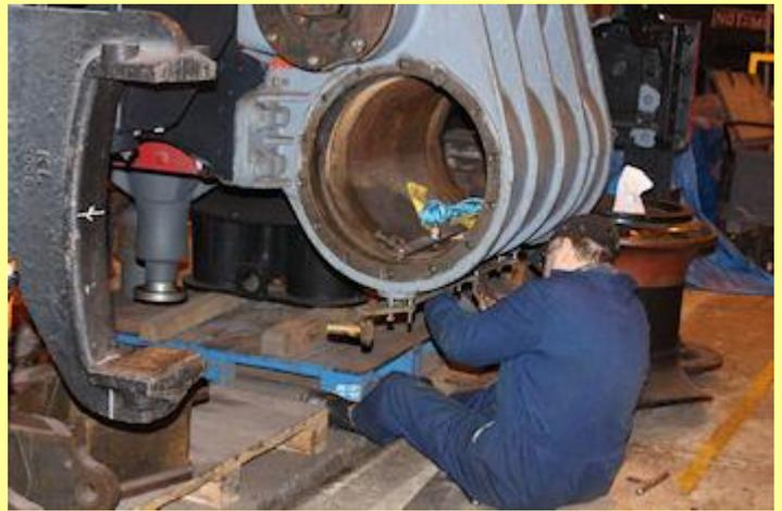
21/12/2013 - Trial fitting bracket for the cylinder blow down cock gear
