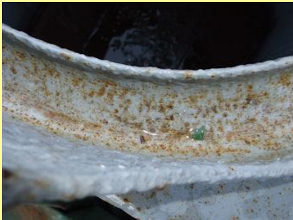
20/12/2014 - mud hole door in its present condition.
